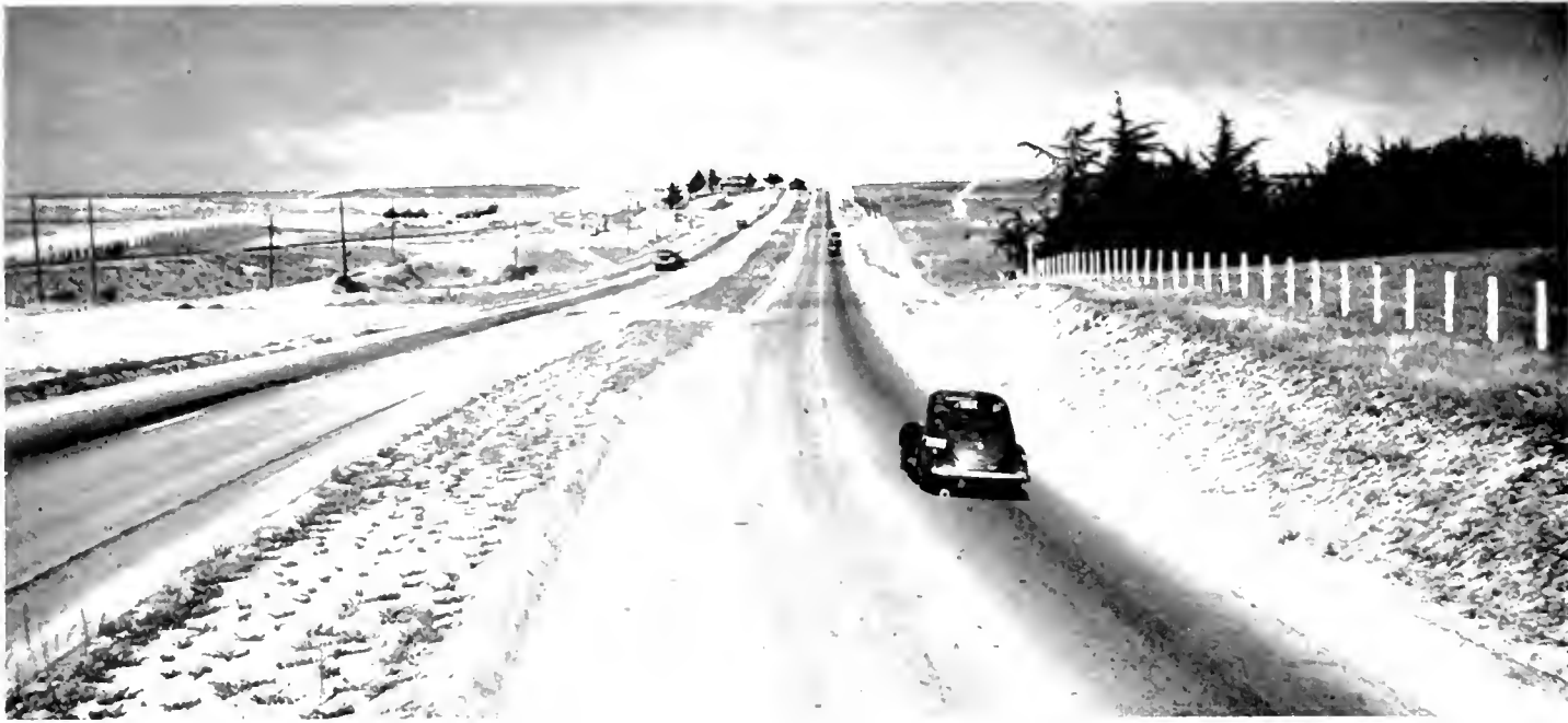
Completed crusher run base with armor coat surfacing between Seaside Junction and North Boundary of Fort Ord
